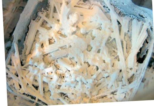
"Weathered" sodium sulfate
