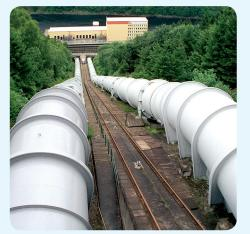
Water shoots down from a high reservoir through these conduits onto the blades of a turbine.
